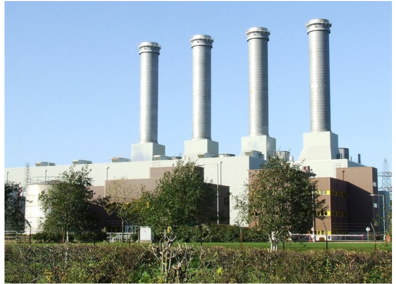
Natural Gas Power Station in North Killingholme , Lincolnshire. Copyright David Hebb
