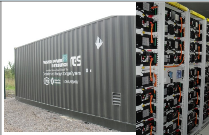
Shipping container containing stacked batteries in Somerset. Copyright Western Power Distribution & British Solar Renewables
